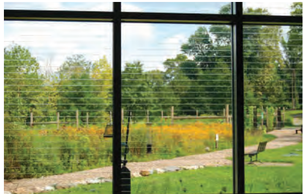
Example of bird-friendly glazing (guideline 28). The pattern shown is etched directly on lower-floor windows to reduce the frequency of bird collisions.
