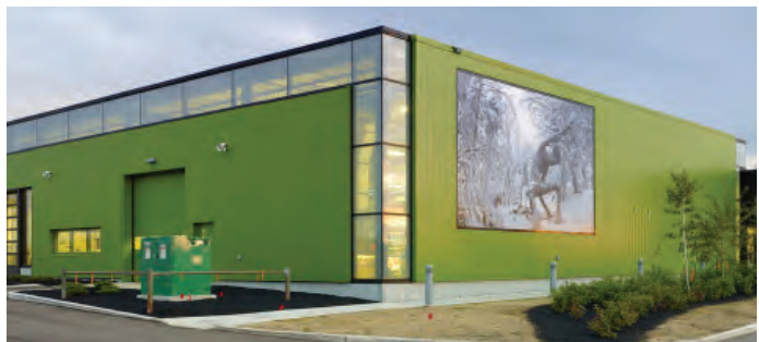
Above two images: Examples of different forms of artistic treatments and landscaping to create visual interest along large expanses of unavoidable blank walls (guideline 26).
