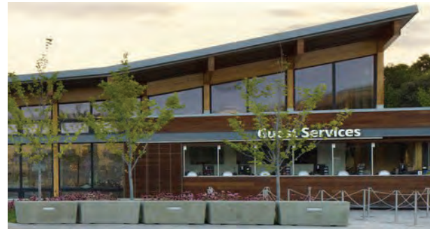
Example of stepped and varied rooflines to develop building form and character (guideline 12).
